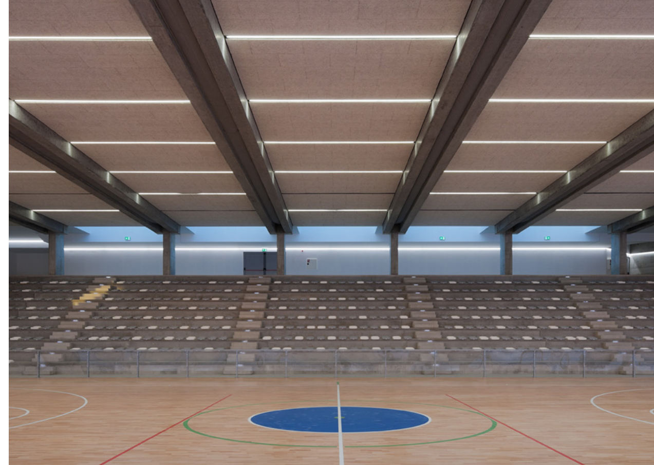
Sport Hall New Sport Hall in Pieve di Soligo Project by Studio Cecchetto
