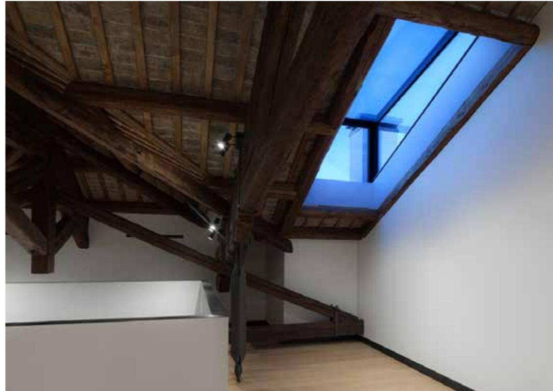
*The attic was created from the garret by modifying the original beams and Glip technical lights are placed.*
